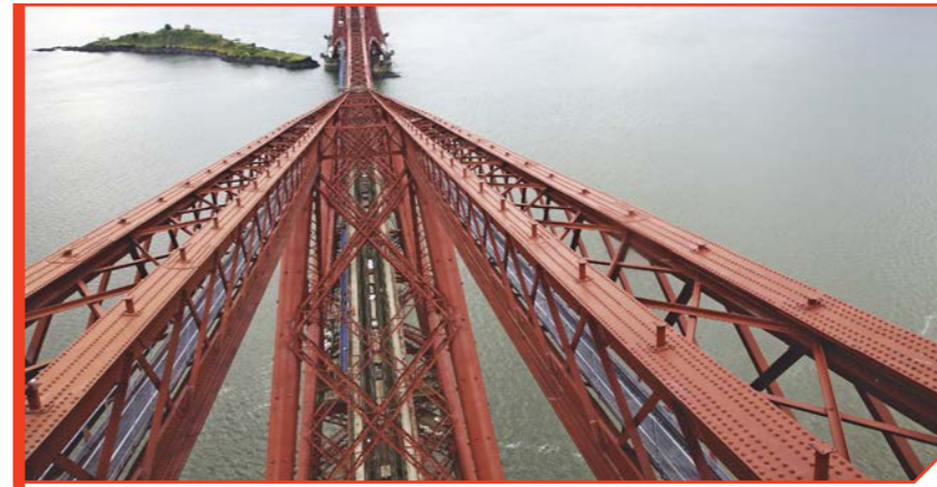
A southerly view from the top of the Fife cantilever, with Inchgarvie island lying just to the east of the bridge. RAIL's Nigel Harris took a once-in-a-lifetime trip onto the Forth Bridge in December 2011 shortly after the decade-long repainting job was completed. You can read the fascinating story of his experience in RAIL 686. NIGEL HARRIS.
