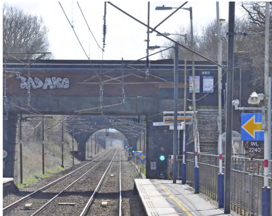
ETCS technology incorporated by Thameslink was tested at the ETCS National Integration Facility at Hitchin and on the Hertford Loop line near Watton at Stone, where ETCS marker blocks can clearly be seen. NETWORK RAIL.
