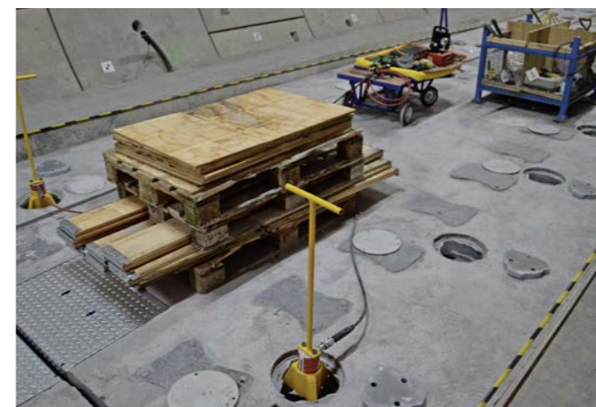
Hydraulic jacks, still in position in Crossrail's eastbound tunnel, that are to be used to raise the FTS to the required height prior to inserting springs and bearings.
