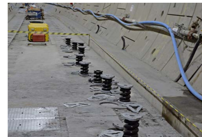
Heavy-duty springs await insertion beneath the freshly set floating track slabs. Each will require 24 hours to settle, and will compress by 10mm under the weight of the slabs.
