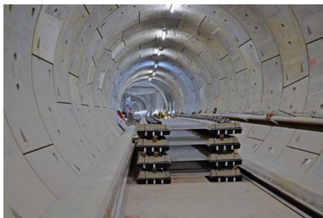
Looking east and back towards Liverpool Street's westbound platform where STS track panels have been stacked, ready to be laid and clipped into position by an MPG. They will then be welded together and concreted into place. Some 70,000 STS sleepers are being used for Crossrail.
