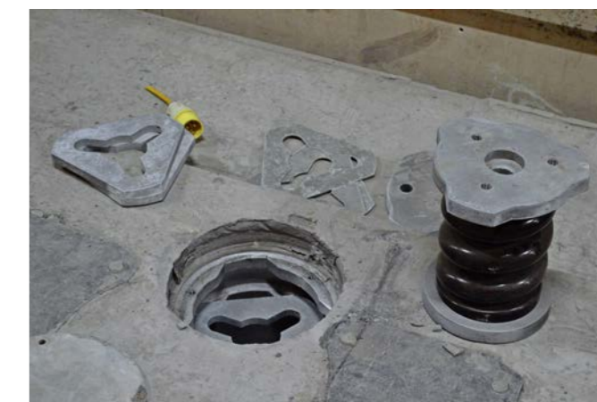
A close-up of the holes that accommodate the springs used for FTS, and the metal shims used to lock them in place.
