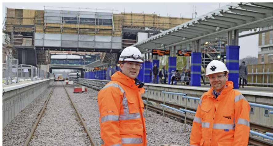
Network Rail's Crossrail Programme Director Matt Steele (left), and Senior Programme Manager Peter Hume inspect the Abbey Wood site on March 24, less than 24 hours before a full line possession commenced to erect overhead line equipment. PAUL STEPHEN.
