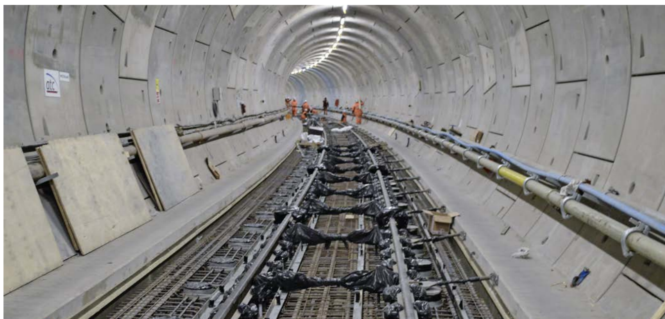
Looking west towards Farringdon in Crossrail's heavy FTS section, and steel rebar is in place ready for that night's Magnadense concrete pour. Up to two 30-metre slabs can be completed during a single shift, with each requiring 45 cubic metres of concrete delivered on site by the grey pipe on the right-hand side tunnel wall. The concrete is pumped up to 900 metres from a shaft on Hayne Street (near Barbican Tube station), as it is too dense for delivery by rail. Concrete pours begin at 1900; grout must first be pumped through the pipe for lubrication before the actual pour can commence. Pumping must be completed by no later than 0100, as Crossrail is limited by a Section 61 agreement with local councils that restricts noise disruption to local residents. The rails on top of the rebar are only temporary, and act as markers for the positioning of steel plates, and the holes needed to insert springs and bearings.
