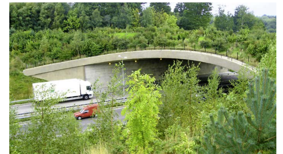
The A21 Lamberhurst Bypass land bridge. This is an example of how integrated design can really work. The landscape acts as a unifying element with the bridge. RICHARD JEVONS/FIRA.
